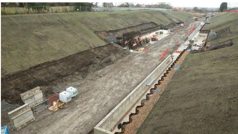
Winslow Station Platforms under construction in December 2021
