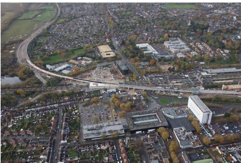
Bletchley Flyover structural competition, November 2021. Image courtesy of Network Rail Air Ops
